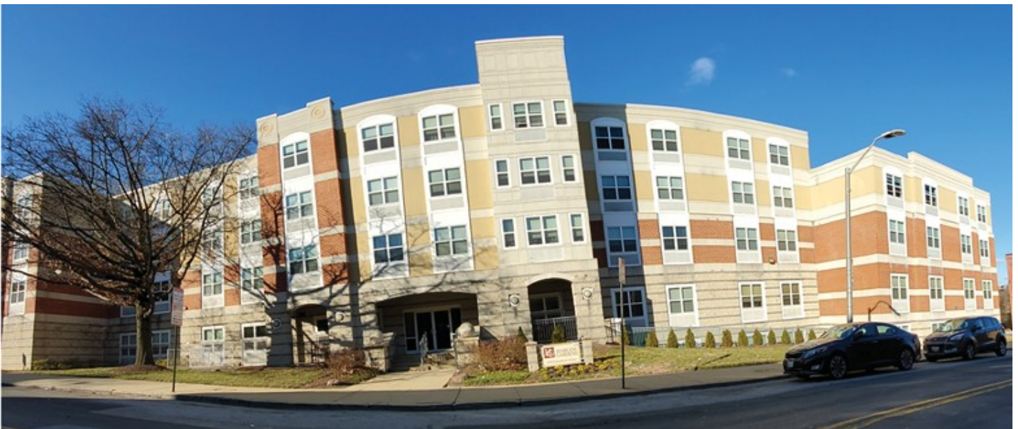
Harlem Park Senior Apartments (with commercial kitchen)
